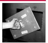
Insert the door into the opening at an angle and then center the door.
