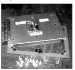
Remove the fasteners and separate door from frame.
