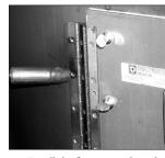
7. Install the fasteners with washers. For hinged door, position hinge on duct wall and plug weld.
